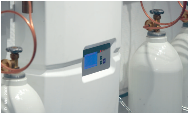
All operational GCS parameters are displayed centrally on the control unit.
