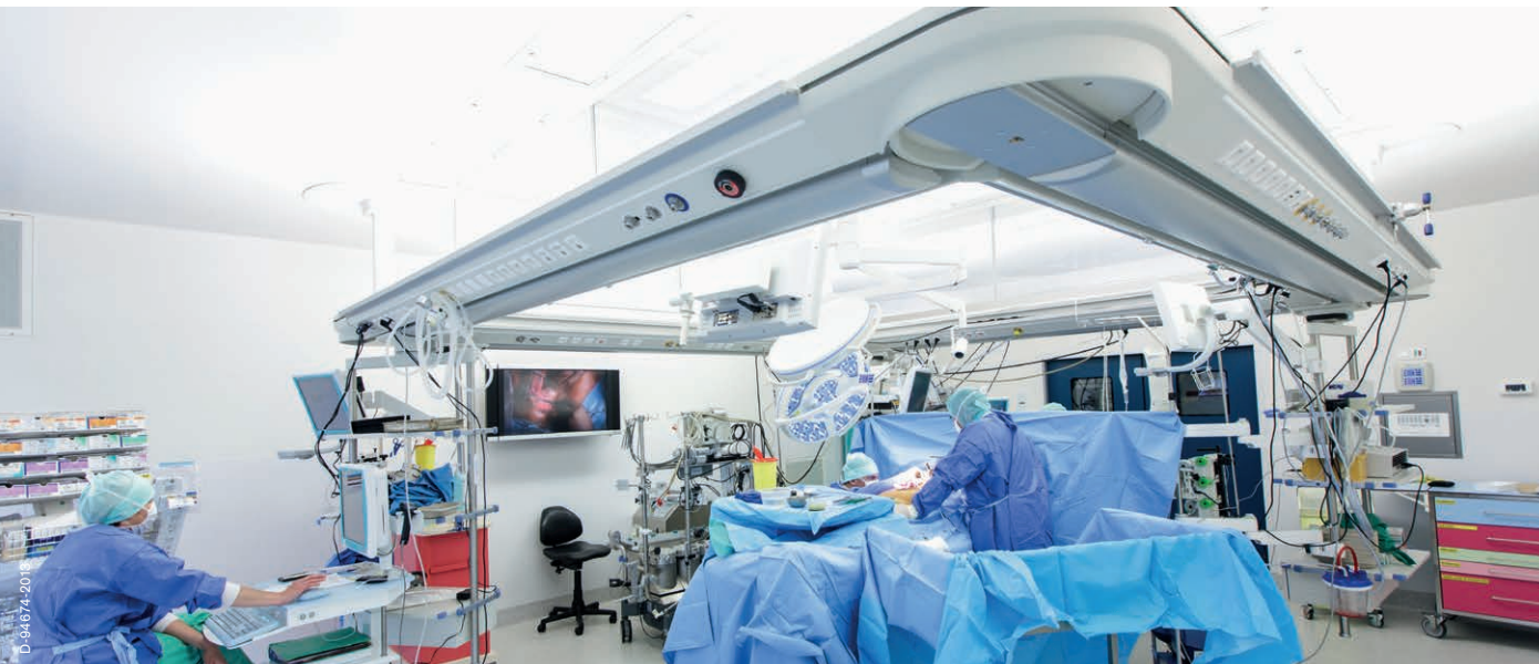
The Opera system enables physicians to completely change the layout of the operating theatre, if necessary.
