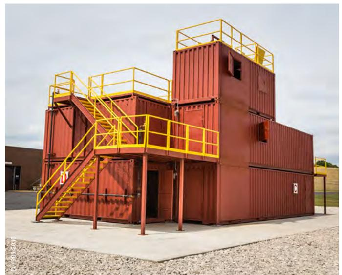
3 level container-based Class A burn structure
