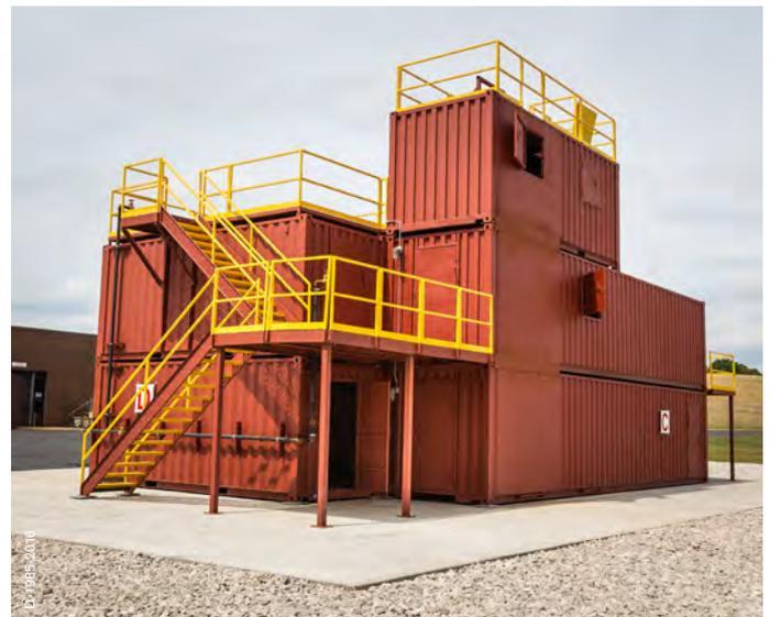
3 level container-based Class A burn structure
